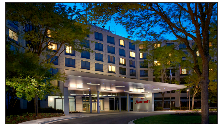
Chicago Marriott Hotel Naperville, IL Six-story | 424 Rooms 275,000 square feet
