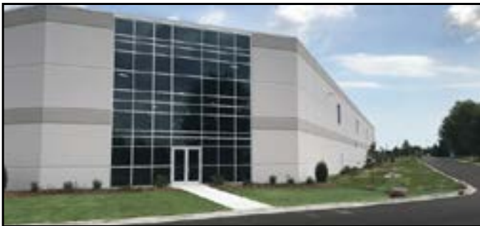
IDI | Pleasant Prairie, Wisconsin Volkswagen Expansion | 90,000 Square Feet Completed Fall 2020 Click HERE for Timelapse Video
