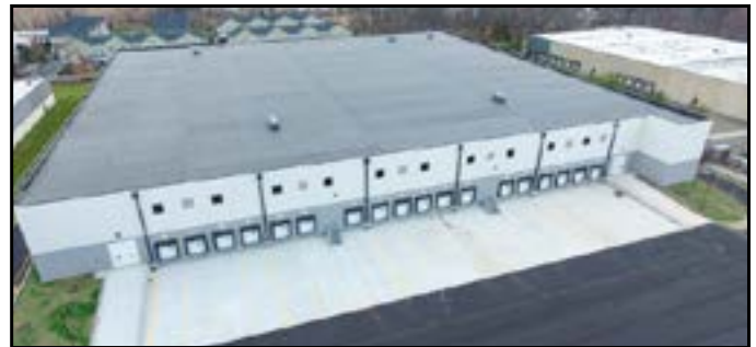
Black Creek Group | Avenel, New Jersey Avenel Business Center | 122,000 Square Feet Completed Fall 2020 Click HERE for Timelapse Video
