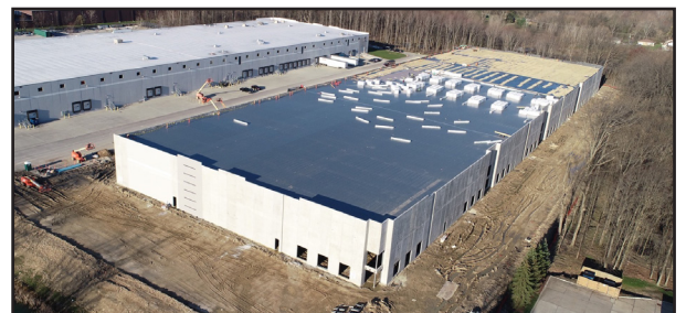
Scannell Properties | Strongsville, Ohio Mills Business Park | 180,000 SF Summer 2020 - Estimated Completion
